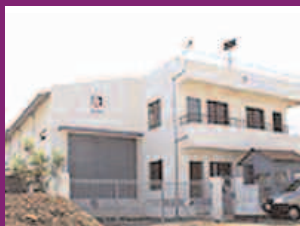
Ross Process Equipment Pvt. Ltd. Pune, India
